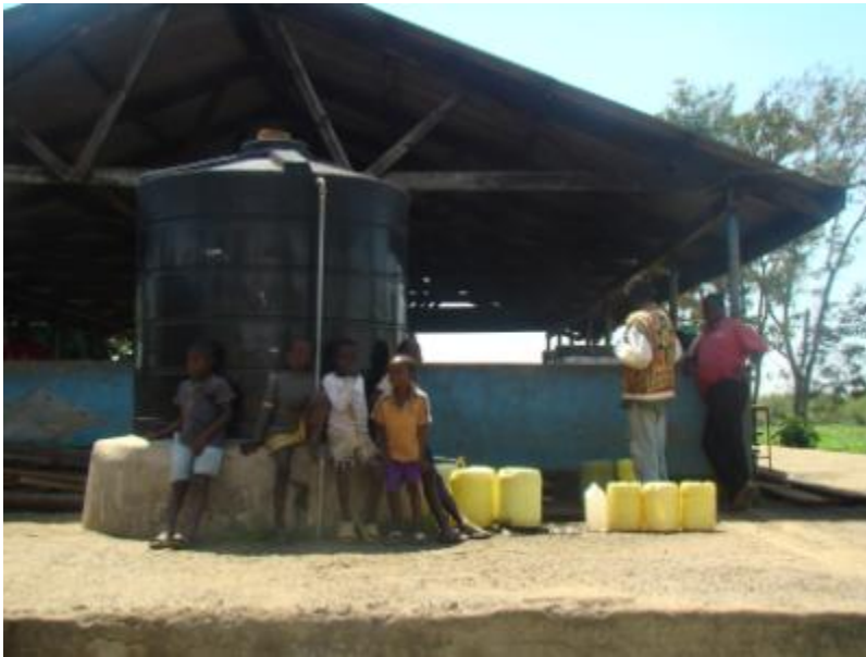
Community-scale water treatment facility in Kisumu (Kenya, September 2008)
