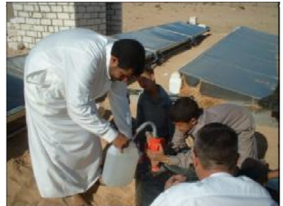
Solar-powered water desalination for rural household use (Egypt)
