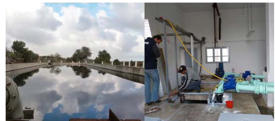
Figure 6: Storage basin of 1,000 m 3 and maintenance of the pumping station in Ouardanine (with permission of O. Mahjoub 2015)
