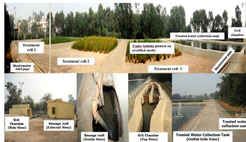
Figure 2: Panoramic view of the proposed (up-scaled) eco-friendly municipal wastewater treatment plant and its components
