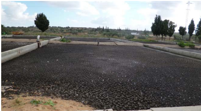
Figure 4: Sewage sludge on drying beds at the WWTP of Ouardanine (with permission of O. Mahjoub 2015)
