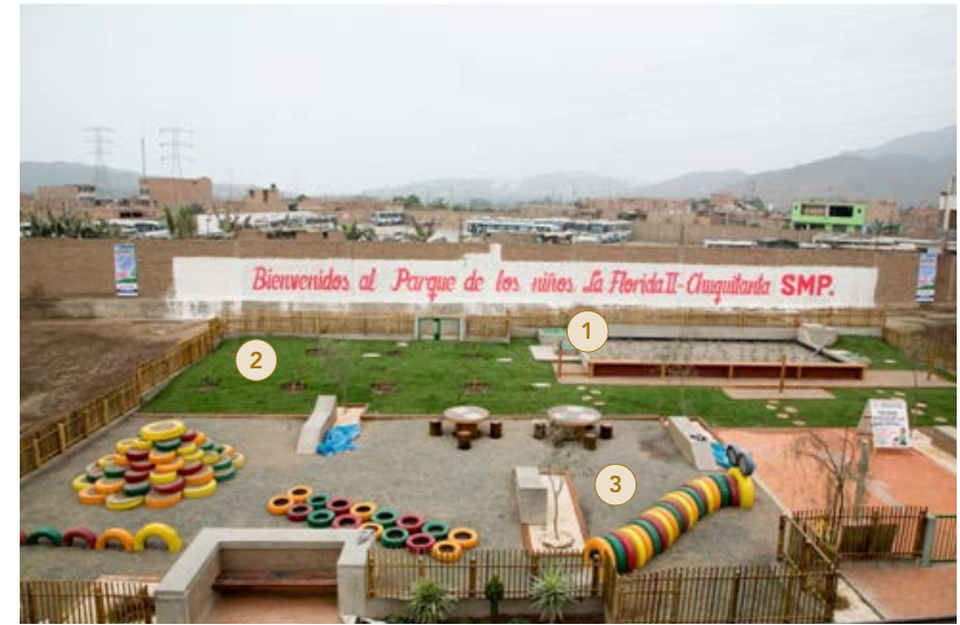
Figure 3: Wastewater Treatment Park – Children's Park on the inauguration day in August 2014, consisting of: 1) treatment system with constructed wetland and reservoir, 2) green recreational area with fruit trees, and 3) play area with dry surfaces (Photo: Evelyn Merino Reyna)
