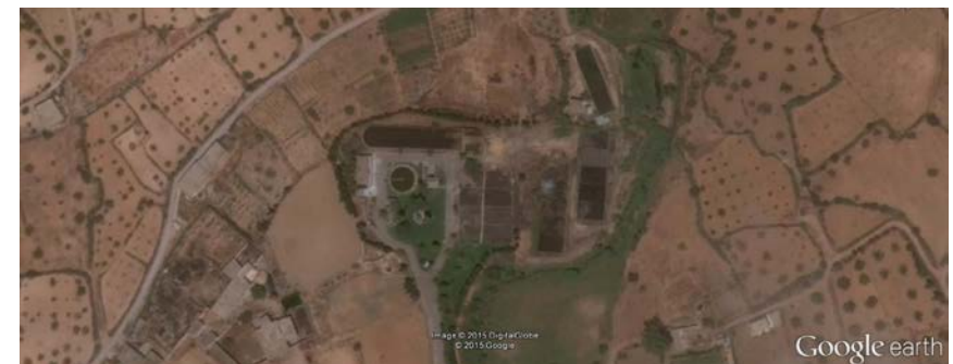
Figure 2: WWTP Ouardanine (Google Earth 2015)
