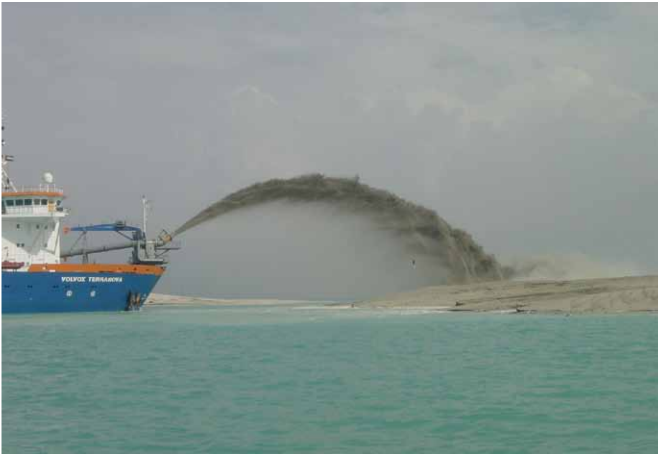
Construction of the majority of coastal developments in the Gulf has relied on locally dredged marine sediments; a dredger adding base material for The World islands, Dubai, UAE, 2006. Credit: Zafar Adeel
