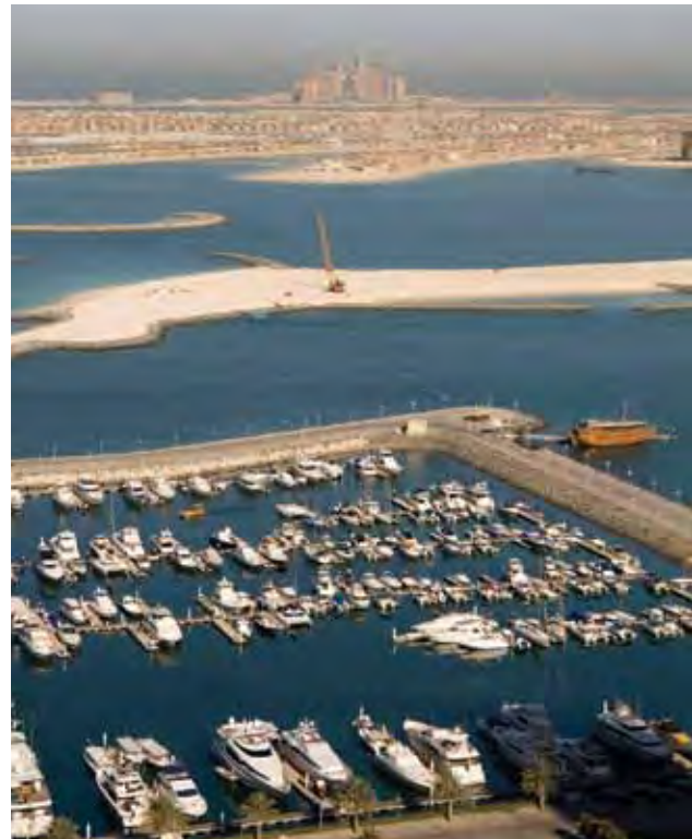
The scale and complexity of coastal development projects in the Gulf region should demand rigorous and comprehensive EIAs. This is an aerial view of a marina and Palm Jumeirah in Dubai. Credit: iStockphoto
