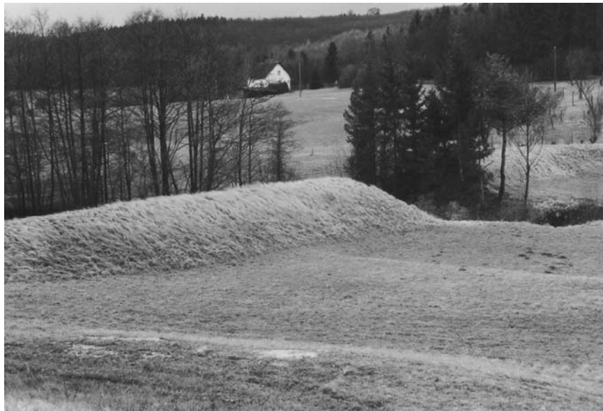
Figure 13.14 An upstream view of Kleinkrottenbach main dam
