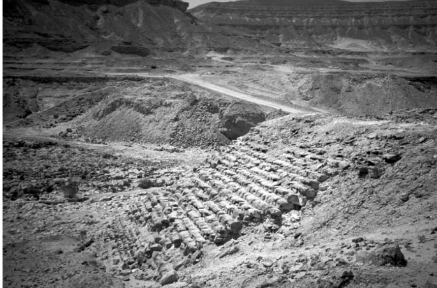
Figure 18.1 Remains of the southern part of the dam
