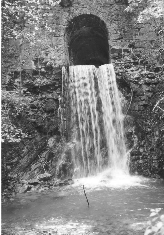
Figure 13.9 A downstream view of the discharge tunnel of Riesenbach Dam
