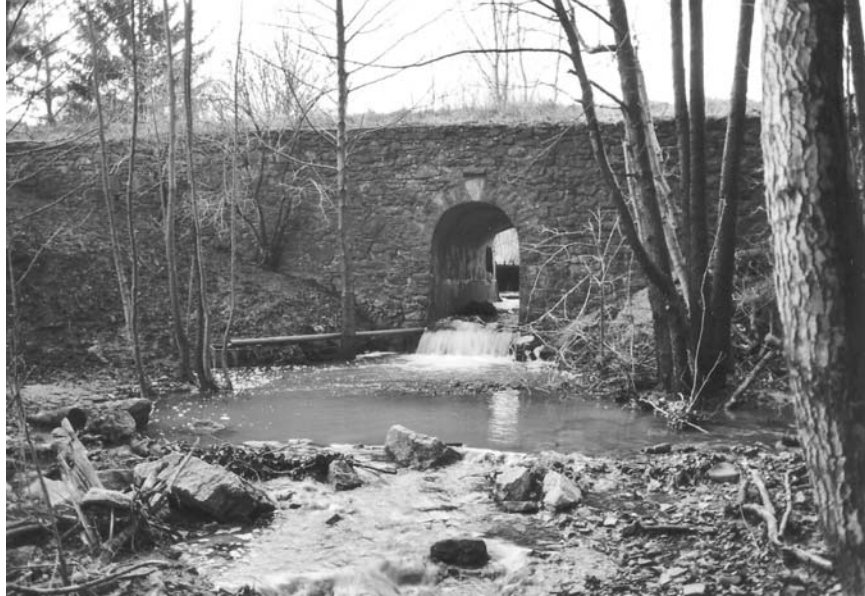
Figure 13.13 A downstream view of the discharge tunnel of Lengbachl Dam
