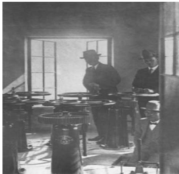
Figure 3.6 Water master in intake tower
