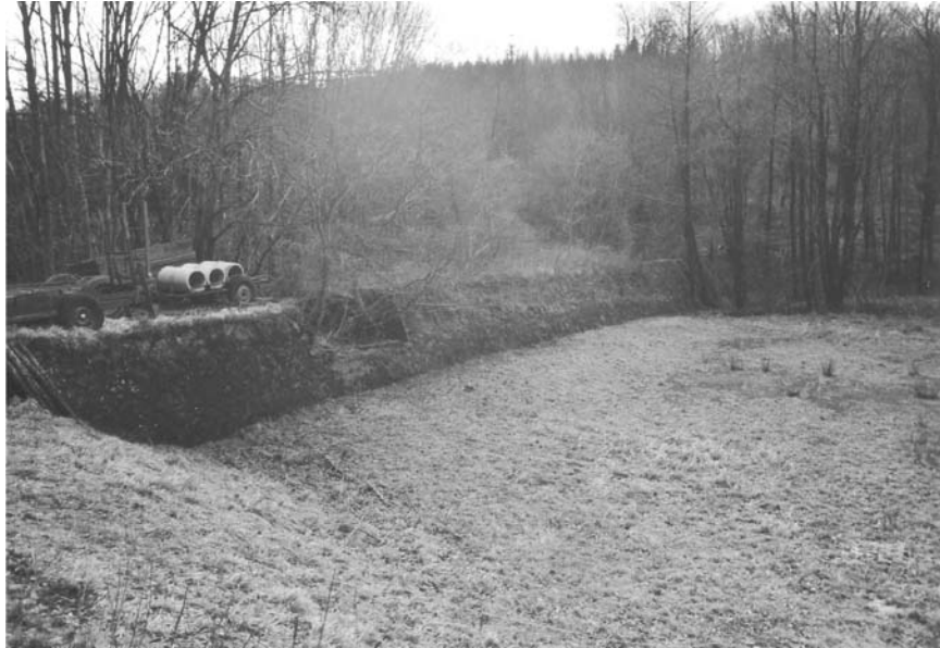
Figure 13.10 An upstream view of Gaisrücken Dam
