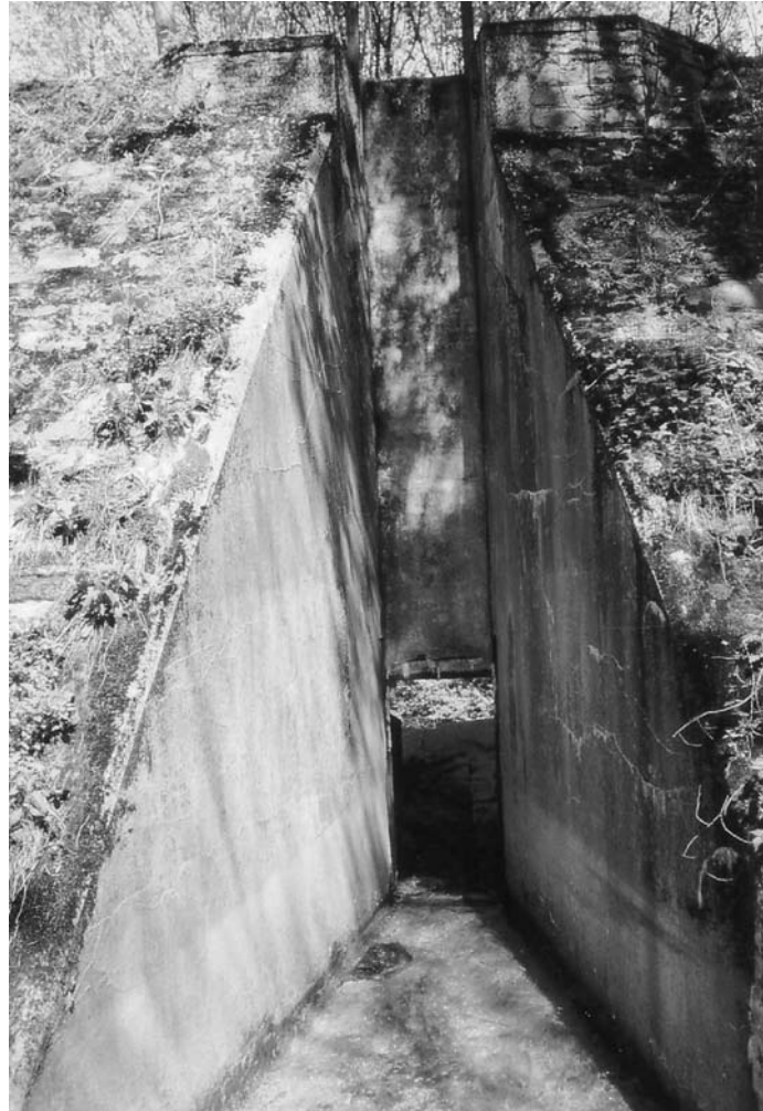
Figure 13.8 An upstream view of the floating gate of Riesenbach Dam
