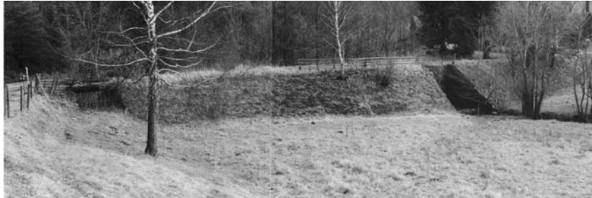
Figure 13.12 An upstream view of Lengbachl Dam
