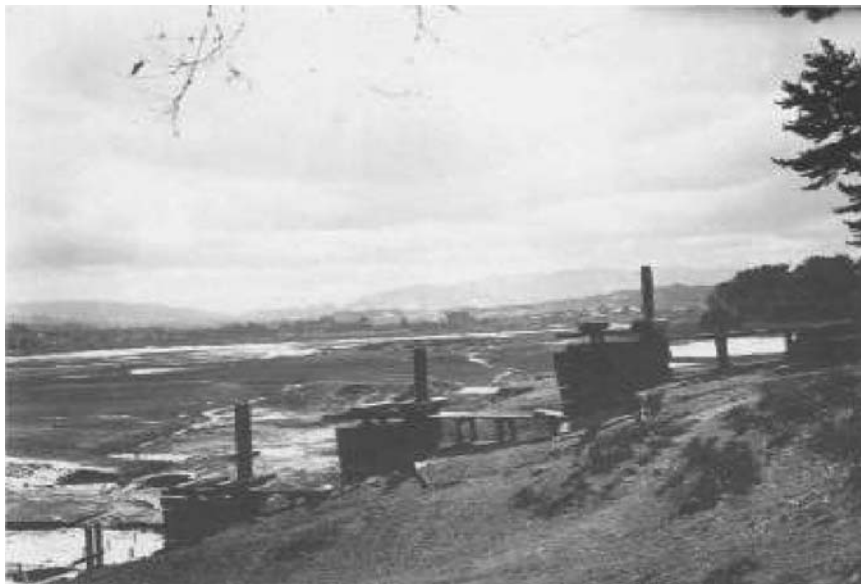
Figure 3.4 Old wooden intake structures
