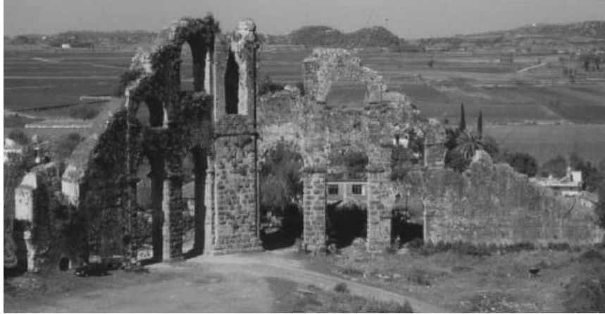
Figure 17.12 South tower of the Aspendos siphon, having a bend of 55 degrees
