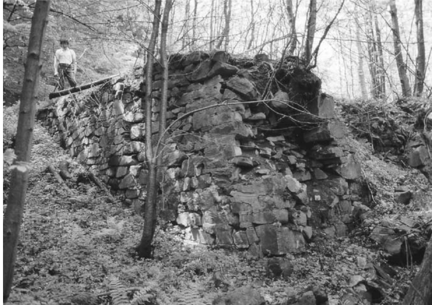
Figure 13.16 The remains of Schöpfl Dam
