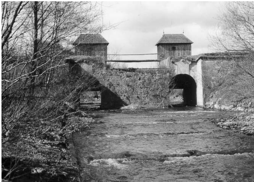
Figure 13.5 A downstream view of Maria Theresia's Fluming Dam
