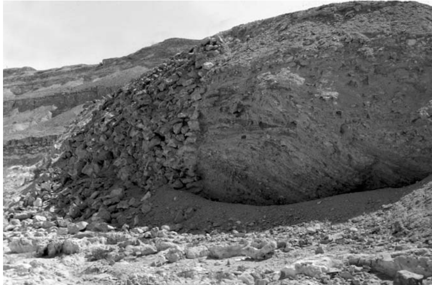
Figure 18.5 Dry wall and rubble fill of the dam
