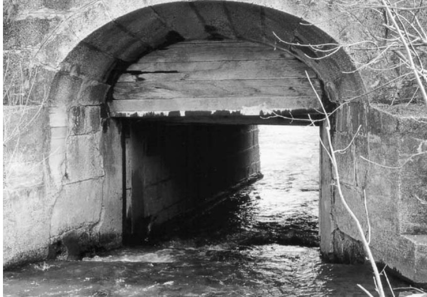
Figure 13.6 An upstream view of one of the renewed floating gates
