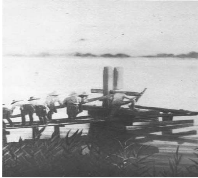
Figure 3.7 Gate-keepers and farmers operating an old intake
