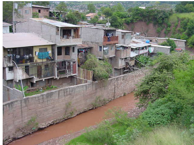
Box 1: Two views of the same trend: whether in large cities or small towns, people think that they can build their house at the expense of narrowing the channels or rivers. However, such measures sooner or later lead to frequent floods in these houses as shown in the upper picture depicting the case of San Sebastian in Guatemala, or to floods in other parts of the city, as displayed in the lower picture from Tegucigalpa, Honduras.
