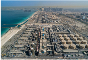
At the Dubai Electricity and Water Authority at Jebel Ali, natural gas is burned to produce electricity and to desalinate seawater for drinking. PHOTOGRAPH BY LUCA LOCATELLI. NAT GEO IMAGE COLLECTION
