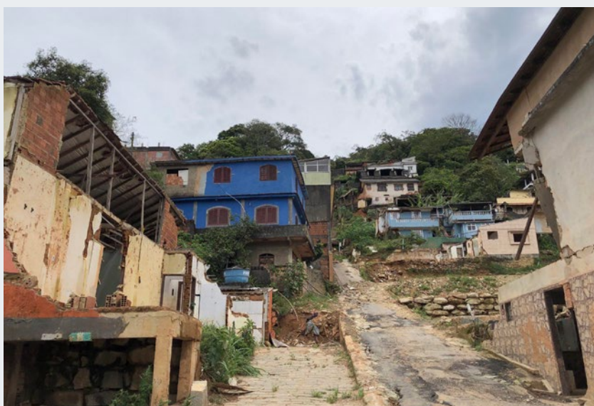
Destroyed houses after heavy rainfall and mudslides from 2022 in Petrópolis, Rio de Janeiro, Brazil. Photo: Klaus/Misereor
