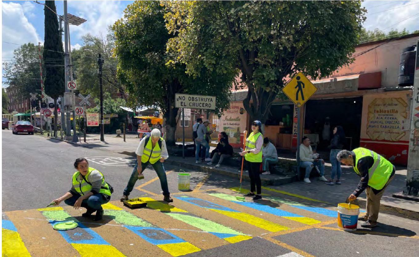
Placement of urban furniture and vegetation in Plaza Revolución and delimitation of crosswalks, August 2023. © WRI México
