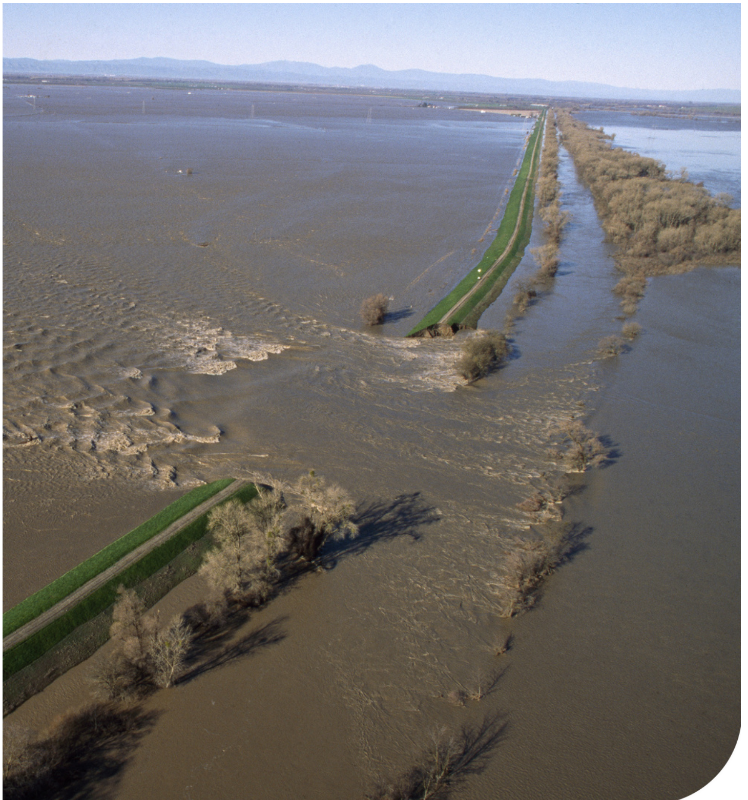
Flood in 1997 forcing a break in a levee, CA, USA. By Dale Kolke, Creative Commons License, Flickr
