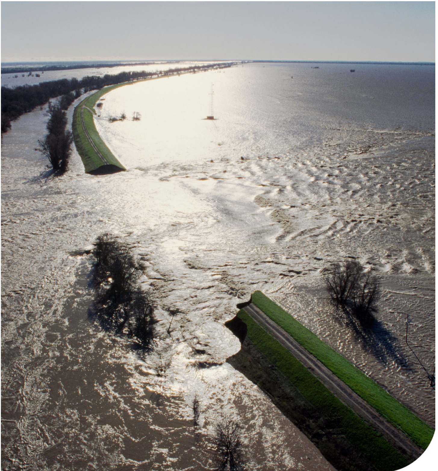
California flood in 1997 forcing a break in the west levee of the Sutter Bypass, CA, USA. By Dale Kolke, Creative Commons License, Flickr
