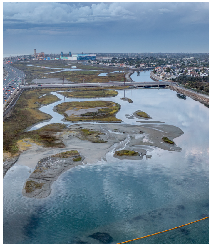
A levee in Santa Ana, CA, USA, with an industrial zone in the right, a coastal estuary in the middle and Pacific Highway in the left. By Amir AghaKouchak
