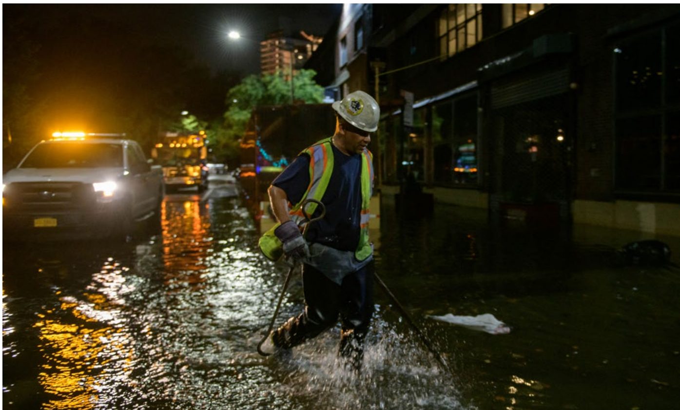
A worker unblocks drains on a street affected by floodwater in Brooklyn, New York early on September 2, 2021, as flash flooding and record-breaking rainfall brought by the remnants of Storm Ida swept through the area. (Image credit: Ed Jones/AFP)
