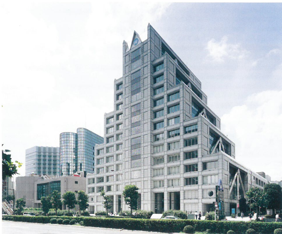
UNU Headquarters building in Tokyo, Japan
