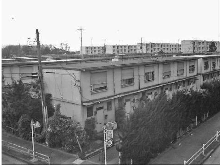
Figure 9.3 An old two-story apartment house ( Source: Photo by the author)
