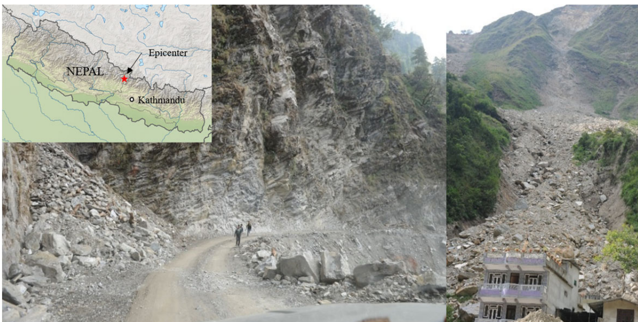
Figure 6 Gorkha earthquake at Nepal on 25 April 2015. a) Rockfall during earthquake at Araniko Highway (Left) (Map from USGS); b) Debris flow during Monsoon season after the earthquake (Right).
