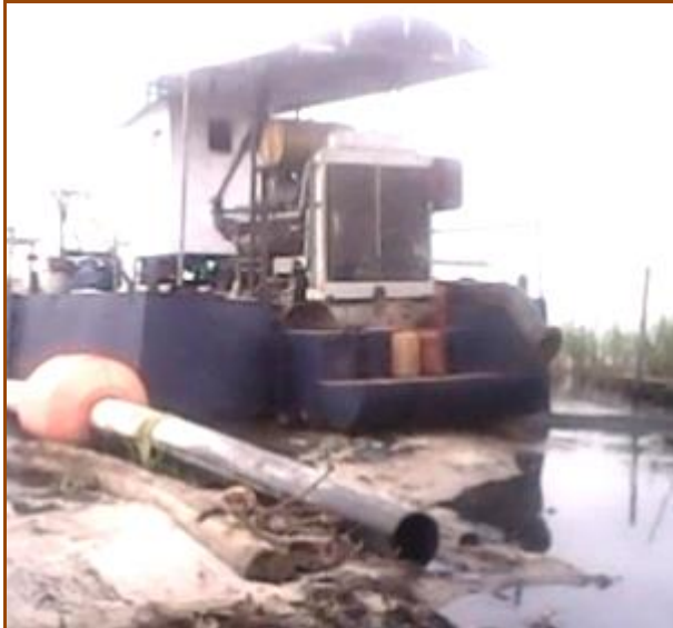
A dredger in action at Epe, Lagos State
