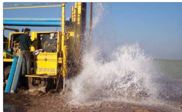
Drilling with hammer in basalts, Guaraní Aquifer System in Uruguay / O. Tujchneider
