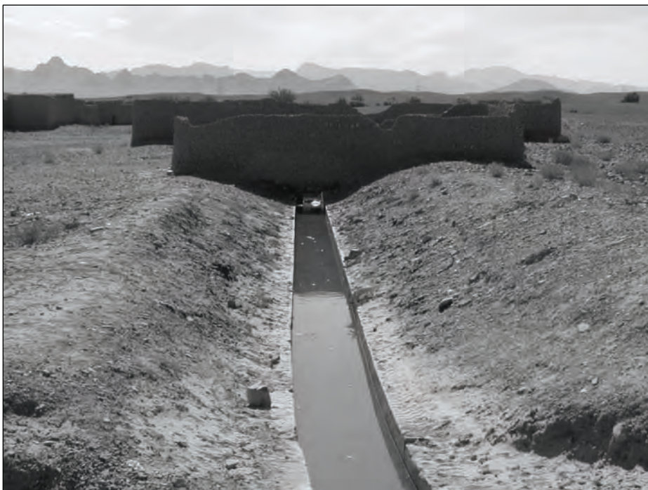
Figure 1. A water channel connecting a karez with the farm.
