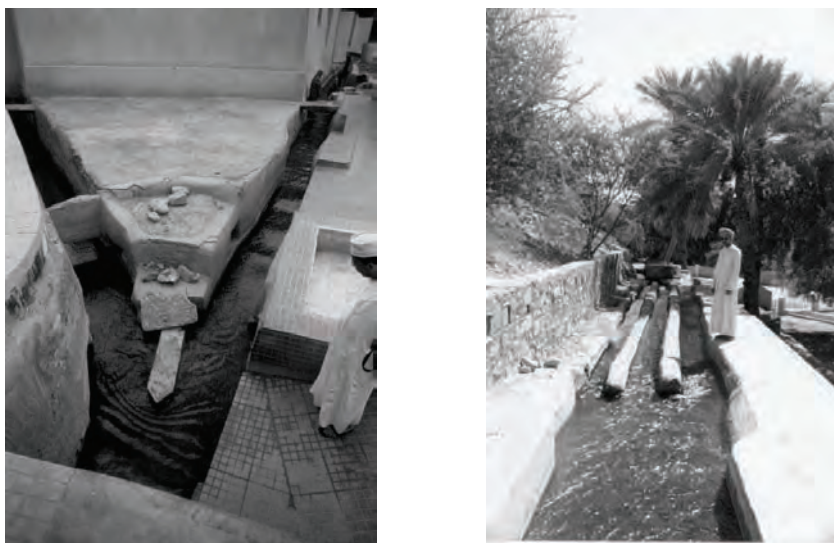
Figure 6. Flow division in aflaj systems.
