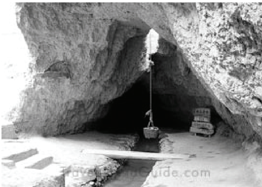
Figure 5. Construction of a karez in Turpan, Xinjiang, China.
