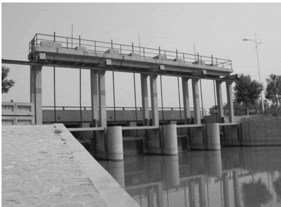
Figure 2: Outlet Gate of Hengshui Lake.
