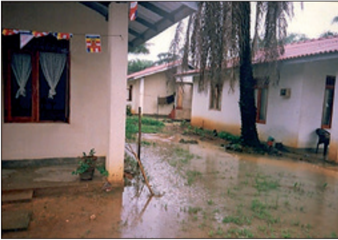
Picture 14: Stagnant rainwater in a house garden at Katupolwaththa Stagnant muddy rainwater as a result of no drainage system at Katupolwaththa
