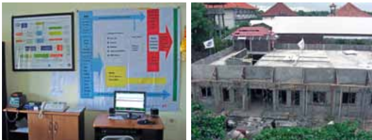
Figure 38: Temporary (left) and new Emergency Operation Centre (right) under construction in Bali
