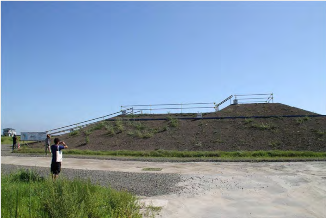
Picture 3: Example for areal elevation according to the reconstruction plan in Yuriage (Photo by authors).
