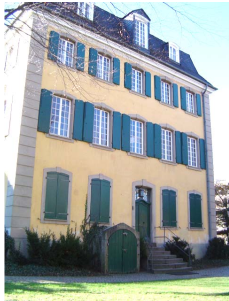
An old building in Beuel incorporating an elevated ground floor to minimize the impacts of floods. Foto: JCV
