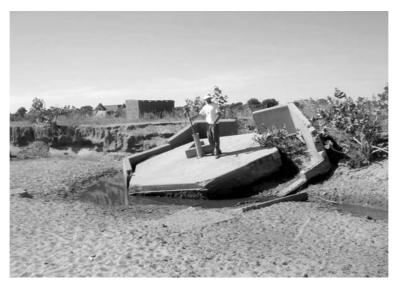
Figure 5: Total collapse of well infrastructure due to seasonal flood erosion, near the village of Abdi in eastern Chad. This can be prevented by locating production wells outside of a wadi, along fractures fed by the wadi's deep reservoir.
